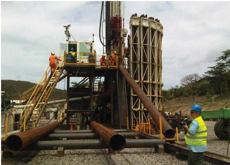
▲ Director of Montserrat Volcano Observatory, Rod Stewart, observing loading of well casing onto drill rig
